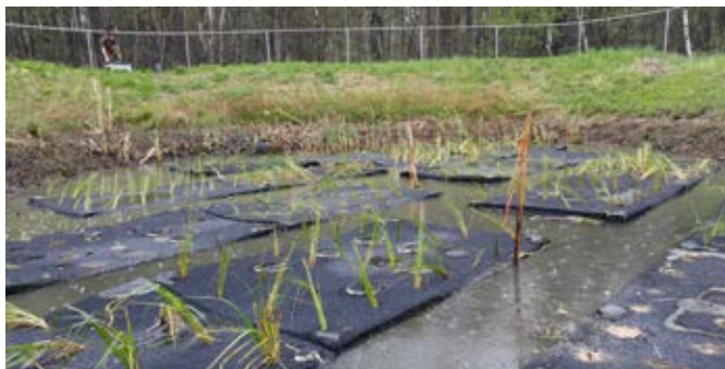
Floating treatment wetland in stormwater pond (Photo: R. Tharp)
