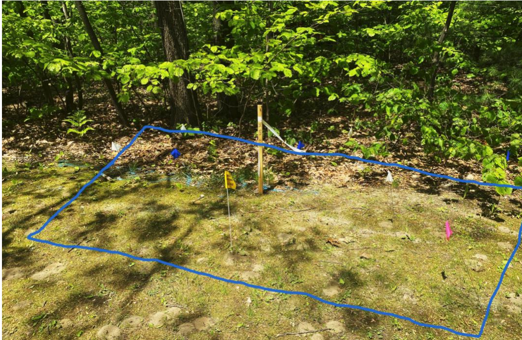
Figure 1. Dig Safe markings on a lawn. The flags indicate the location of utilities. The box outlines the area of interest.
